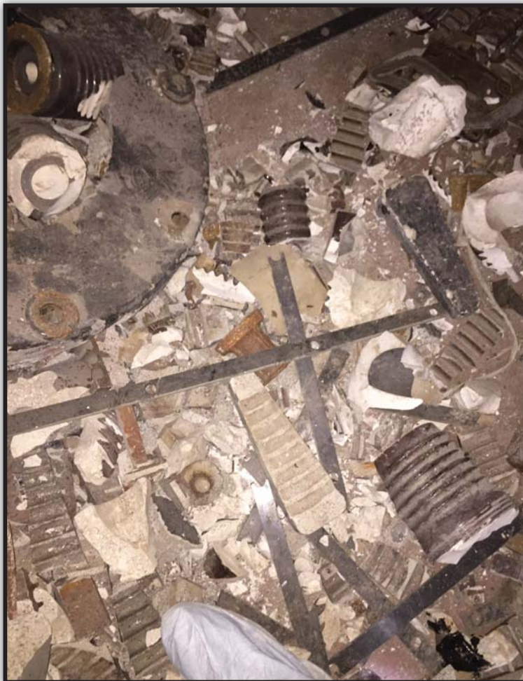
PHOTO 10. English Station - Second Floor, Switch Cell Area.
