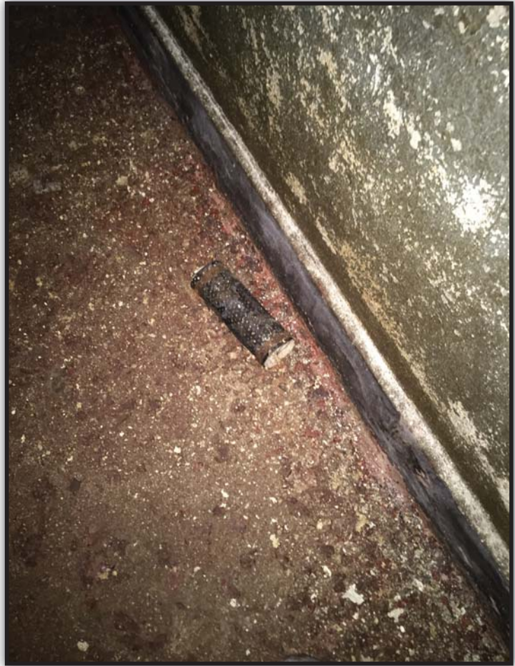
PHOTO 7. English Station - Second Floor, Switch Cell Area.
