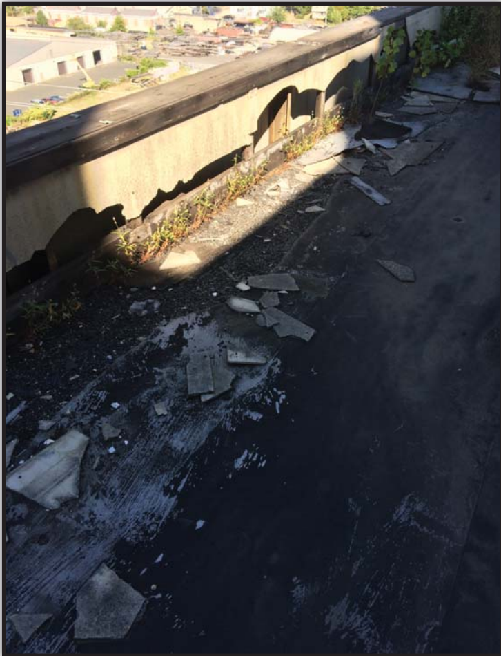
PHOTO 8. English Station - roof above northeast corner of high pressure boiler area.
